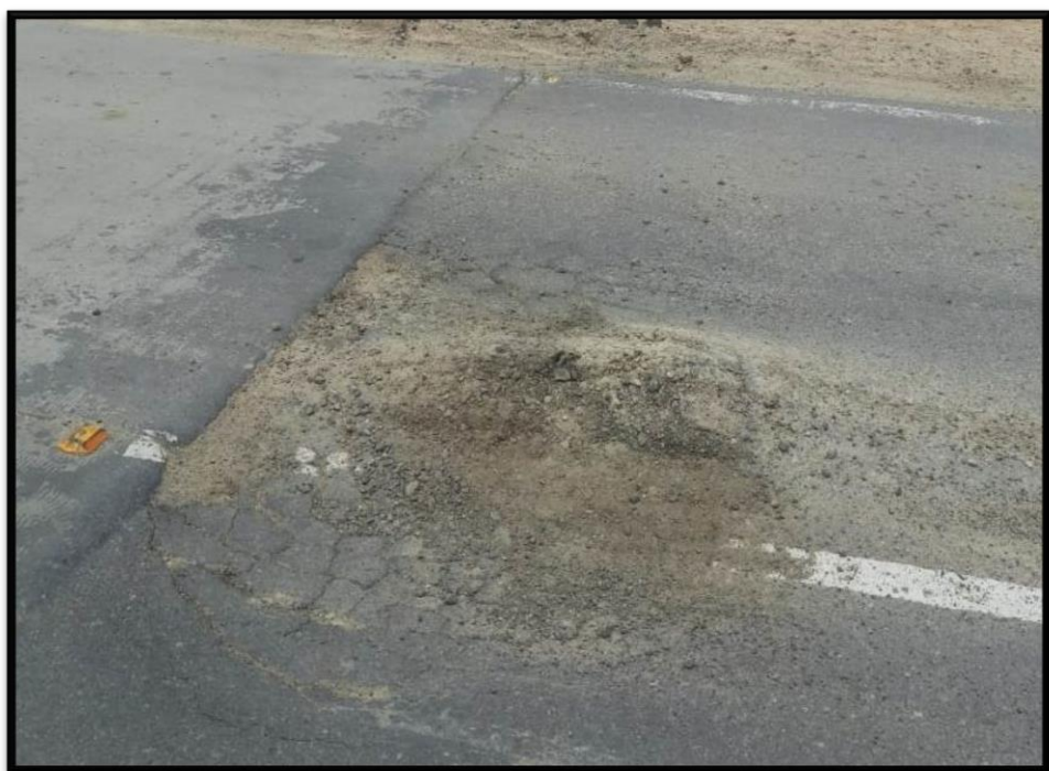
Image 6: Pits on the road
