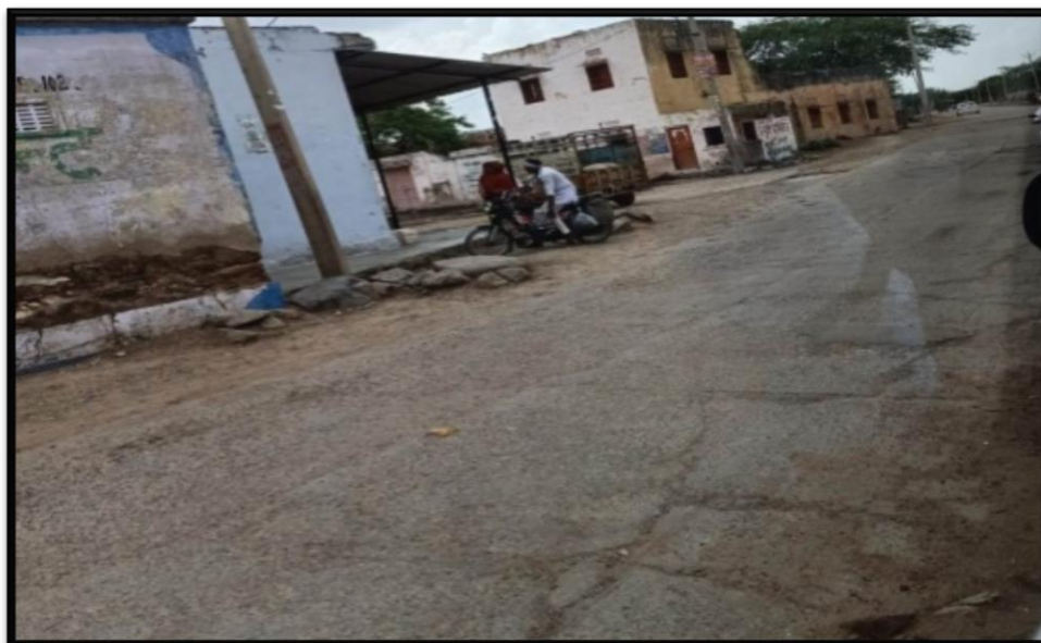
Image 4: Unconstructed stretches of the road
