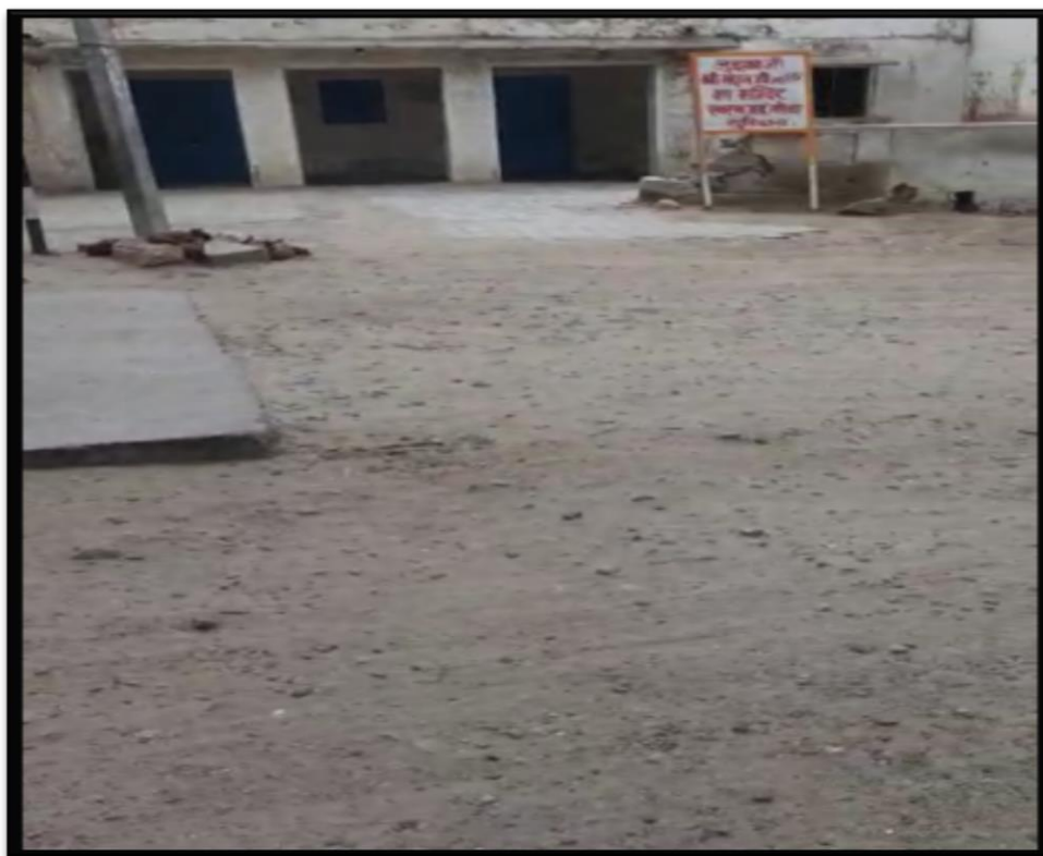
Image 3: Unconstructed stretches of the road
