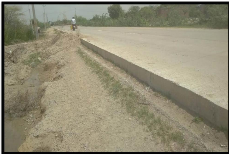
Image 1: Missing interlocking blocks/GSB shoulder/drain
